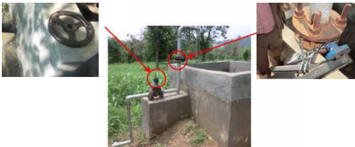
Fig. 4.3 Lock System for Valves in the Pilot Area
