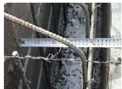
5. Photograph Recording (Cover and formwork spacing)
