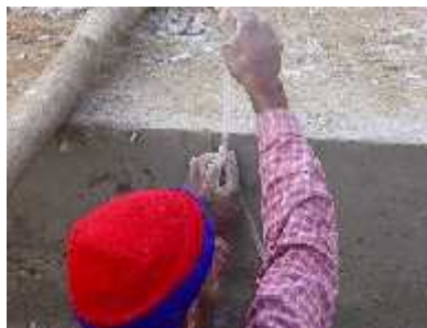
Direct Measurement of elevation by water tube
